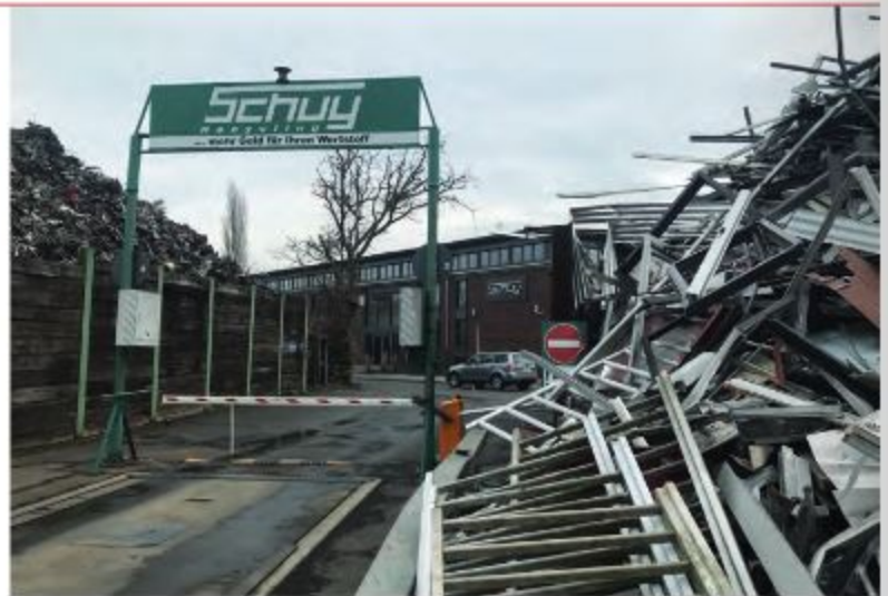
EUR 4 million were invested in the complex (background) that is currently the company's stylish headquarters and office building.
